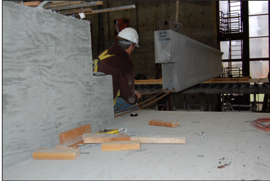
Figure 3.19: Pushing the Strands through the Girder
