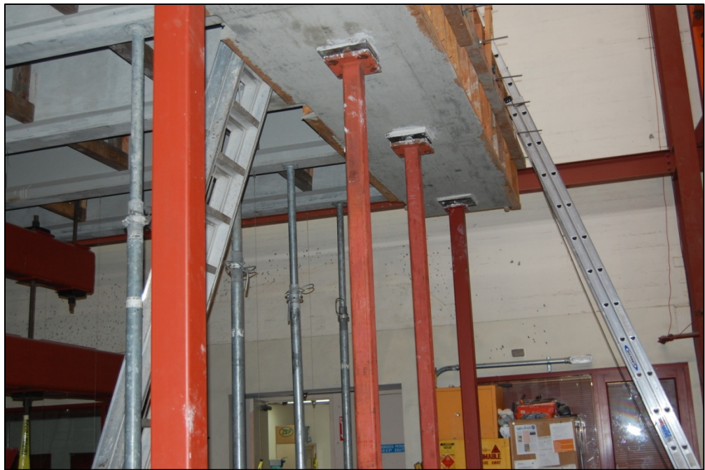
Figure 3.15: Temporary Support System Used Under Each Abutment
