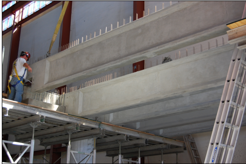
Figure 3.13: Installation of Southern Girders
