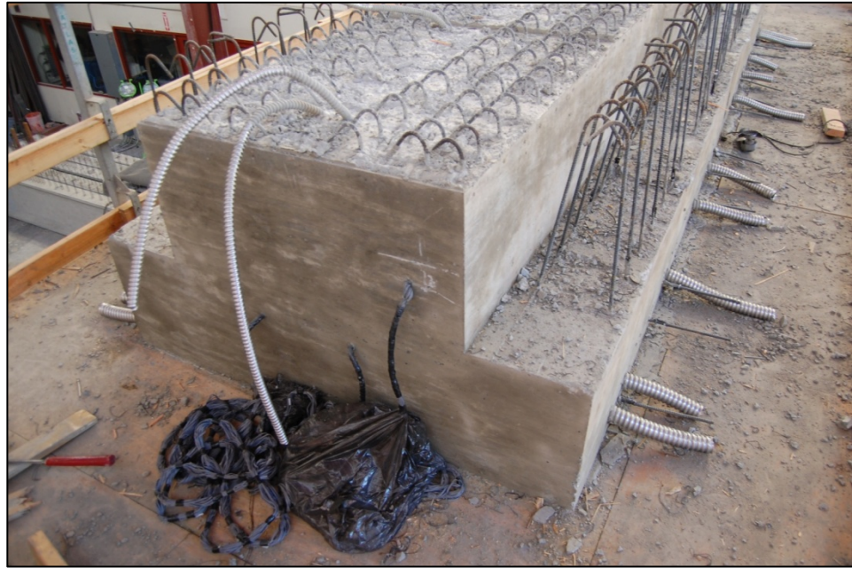
Figure 3.12: Completed Bent Cap Construction on Top of Column
