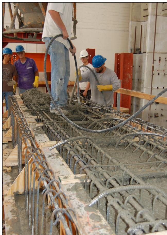
Figure 3.16: Casting of the Bent Cap
