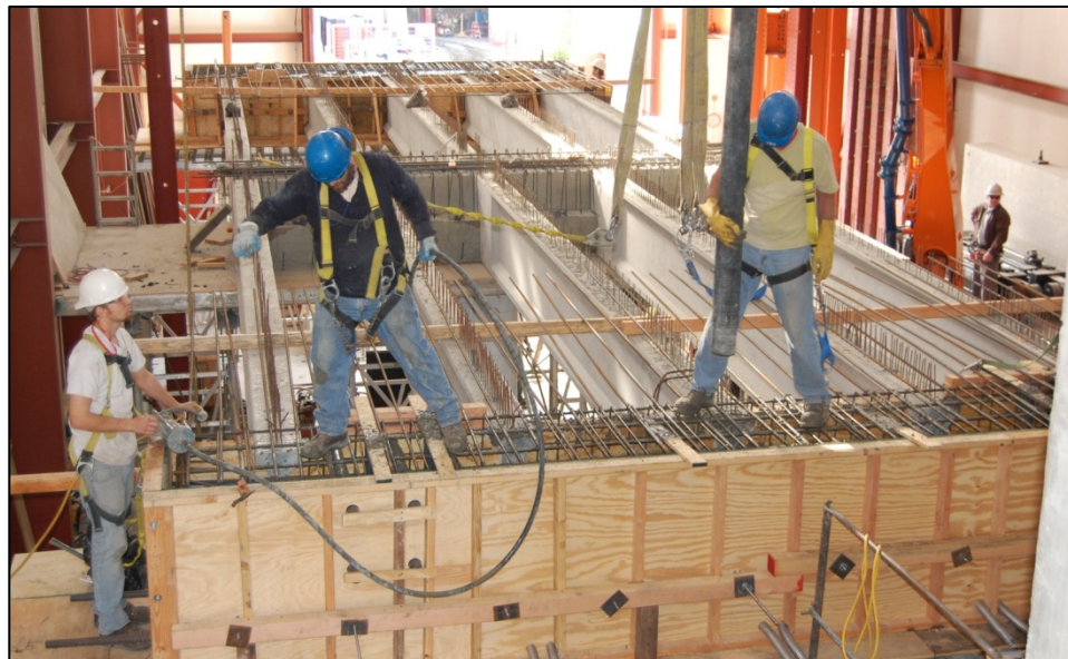
Figure 3.14: Casting of the North Abutment
