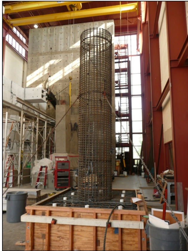
Figure 3.10: Completed Column and Footing Cage
