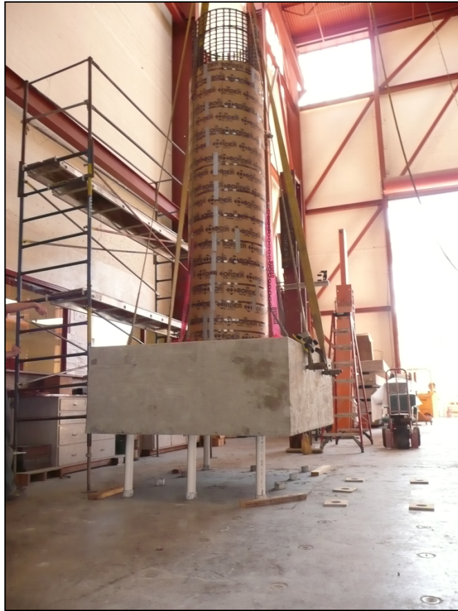
Figure 3.11: Replacing the Column and Footing
